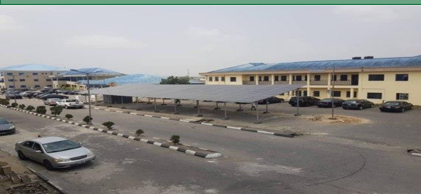
50 KW solar system at Federal Medical Center Yenagoo, Bayelsa State
