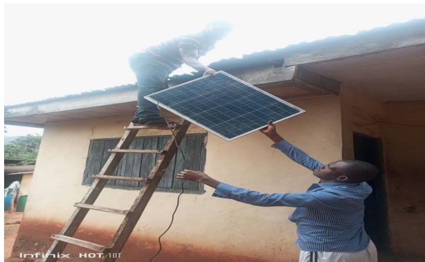
Installation of SHS systems
