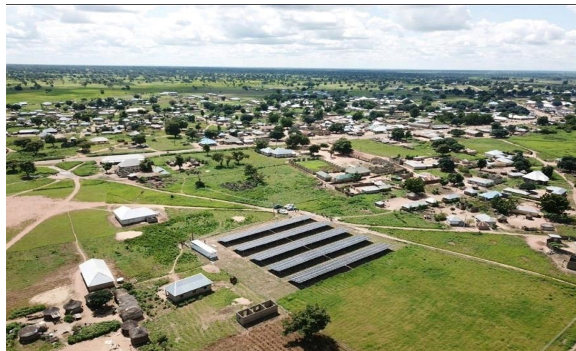
234kWp mini-grid, Shimankar, Niger State
